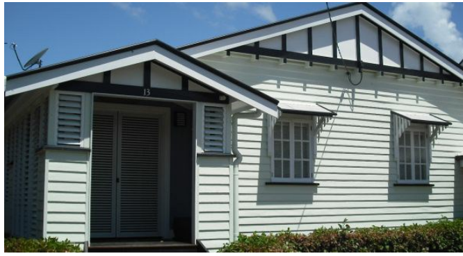
Figure SC6.2.3.19 Illustrates traditional use of timber chamferboard on external walls
