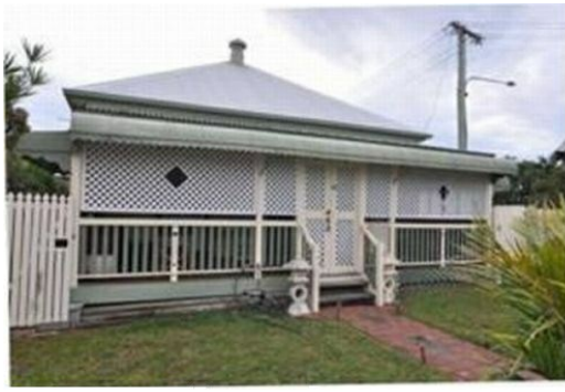
Figure SC6.2.3.7 Illustrates an example of a front verandah, semi enclosed with screening and a door
